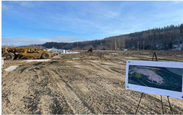
Site grading at Prince George (2.4 EH/s, 85MW)
