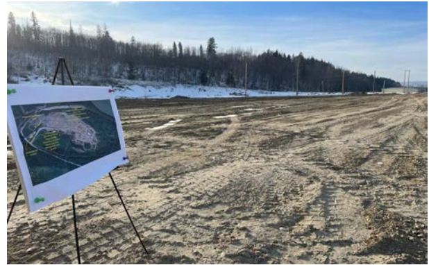
Site grading at Prince George (2.4 EH/s, 85MW)
