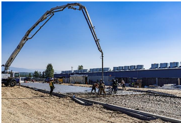
Mackenzie – concrete slab pour at the fourth data center building (20MW)
