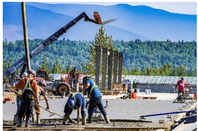
Mackenzie – erection of structural steel at the fourth data center building (20MW)
