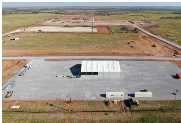
Childress – aerial view of the warehouse, substation and data center areas
