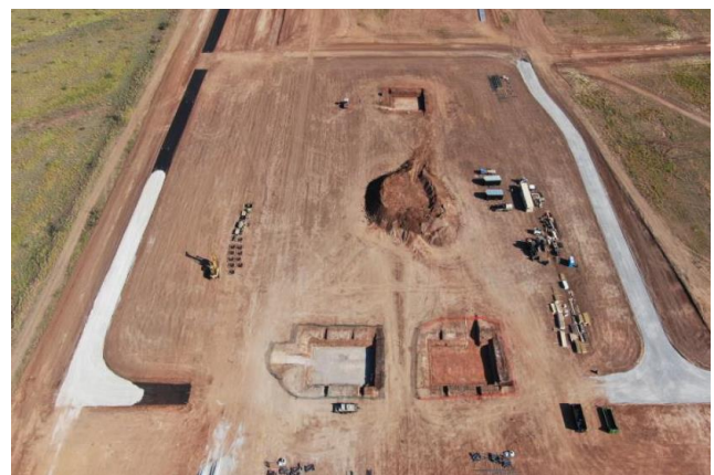
Childress – aerial view of substation foundation preparations
