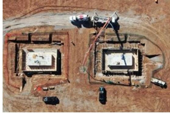
*Childress – aerial view of the bulk 600MW substation foundation preparations*
