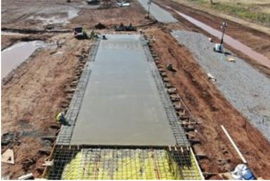
*Childress – concrete slab pour at the first data center building (20MW)*
