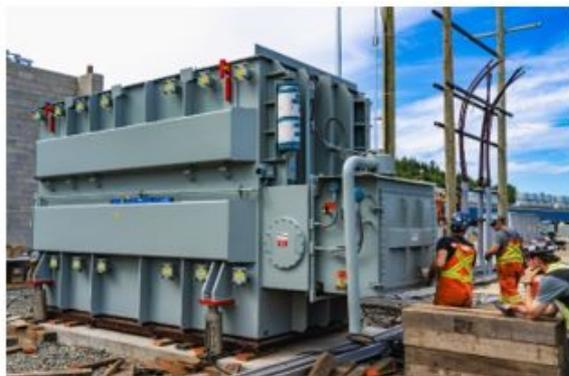
*Prince George – 69kV high voltage transformer being positioned*
