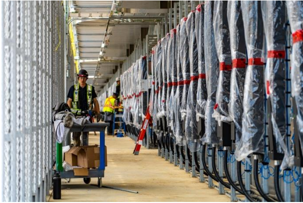
Prince George – PDUs being installed
