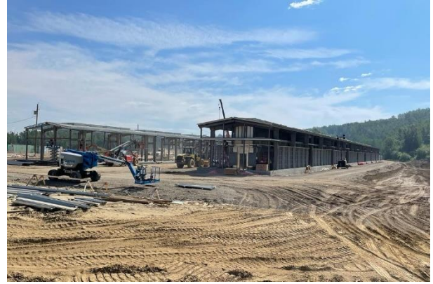
Prince George – data center construction in progress
