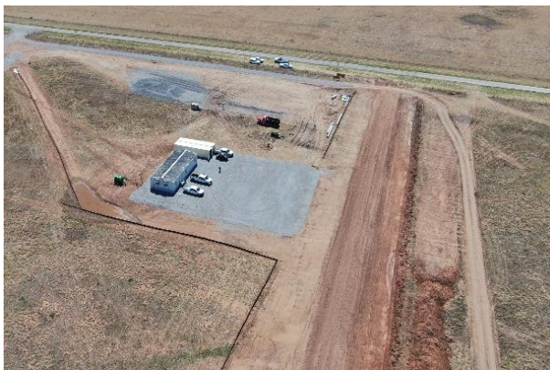
Childress – site construction office and entrance
