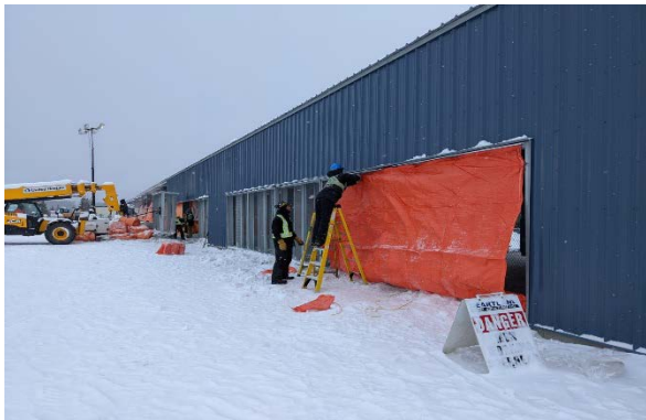
Construction at Mackenzie (1.5 EH/s, 50MW)
